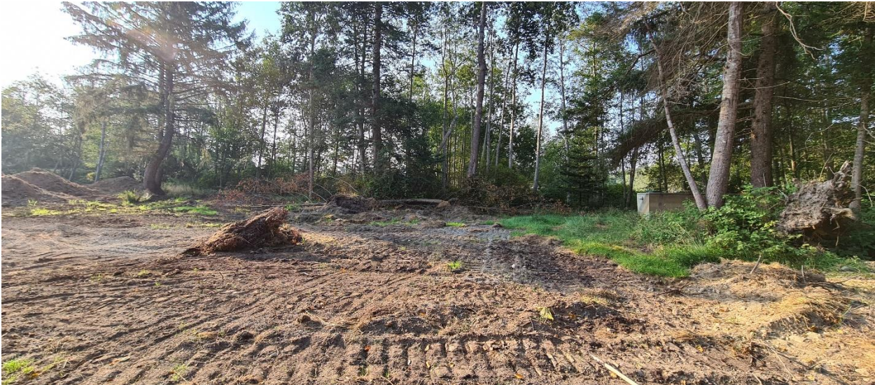
Rear area of fill
