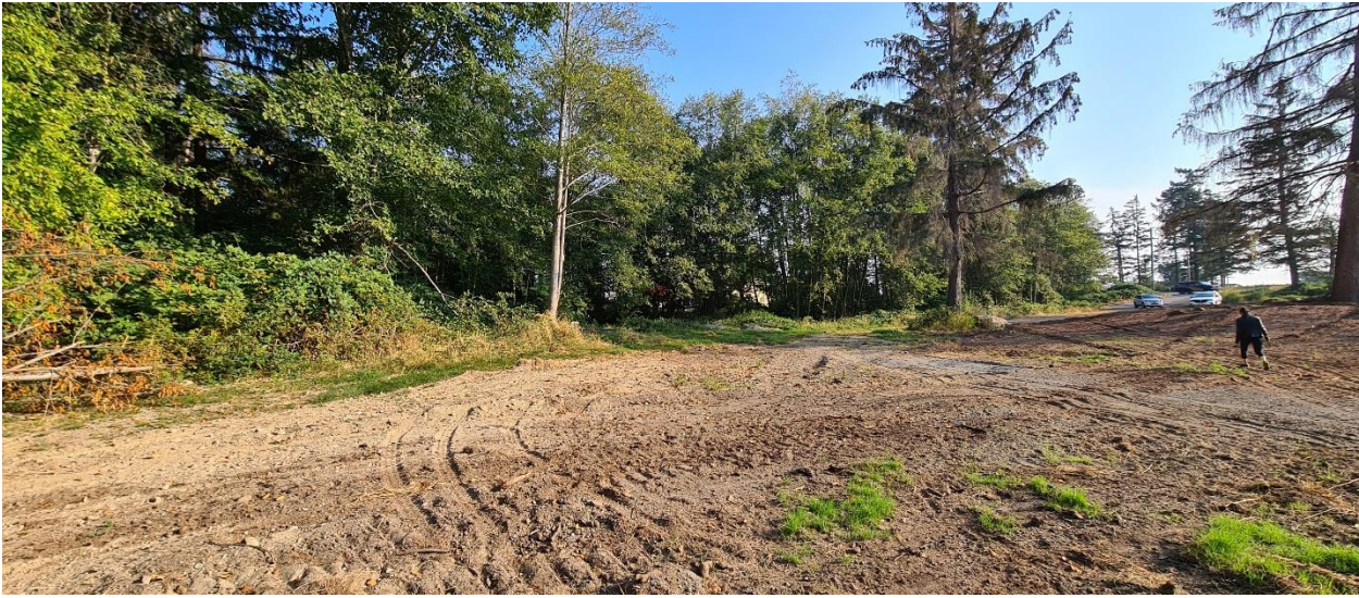
Fill area looking east
